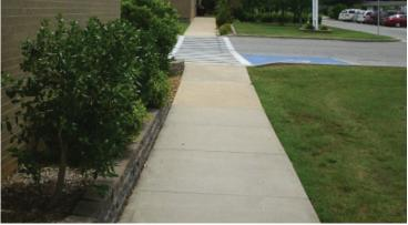
Materially, sidewalks on the campus are primarily concrete with a gray natural finish. Coordinating concrete curbs, some painted to designate fire zones or loading, are in place to transition to driving surfaces. Landscape edging is set with either a raised concrete lip or dark gray/brown split faced edging blocks. Dark asphalt covers the parking areas while crosswalks are painted onto paved surfaces.
